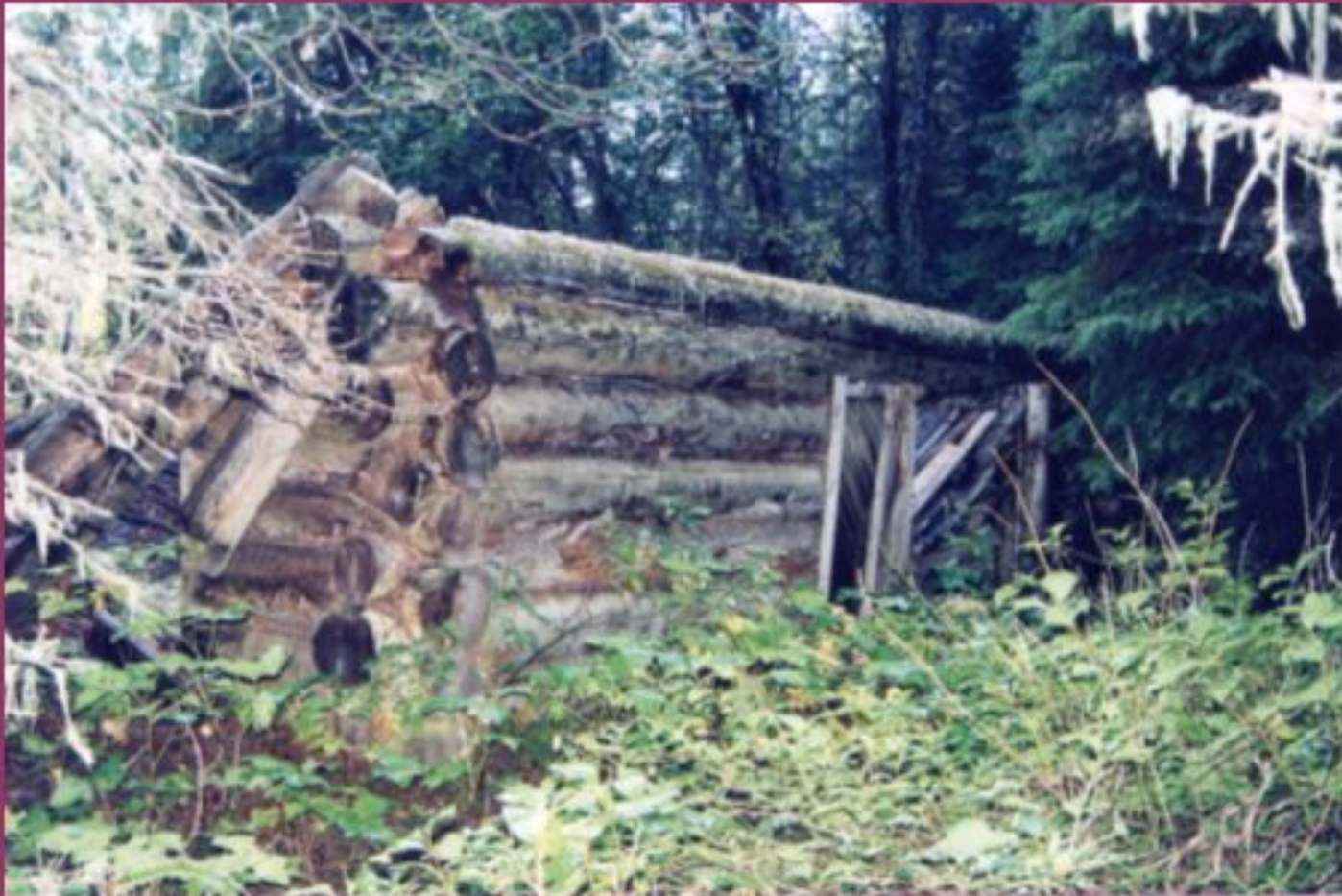
What is left of the Cameron homestead house
