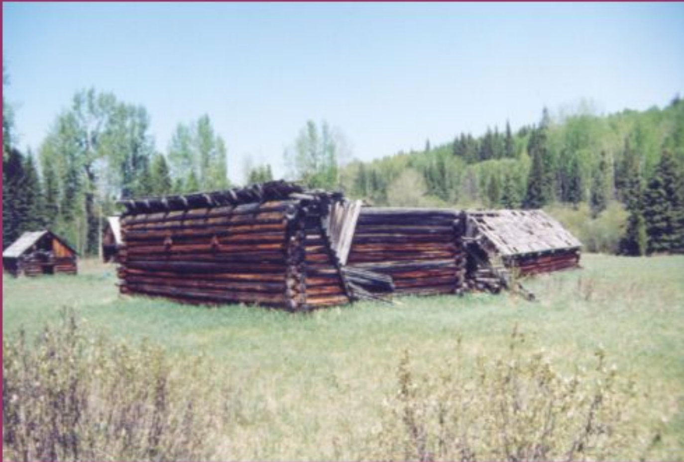
Tereschuk homestead with barn roof caving in
