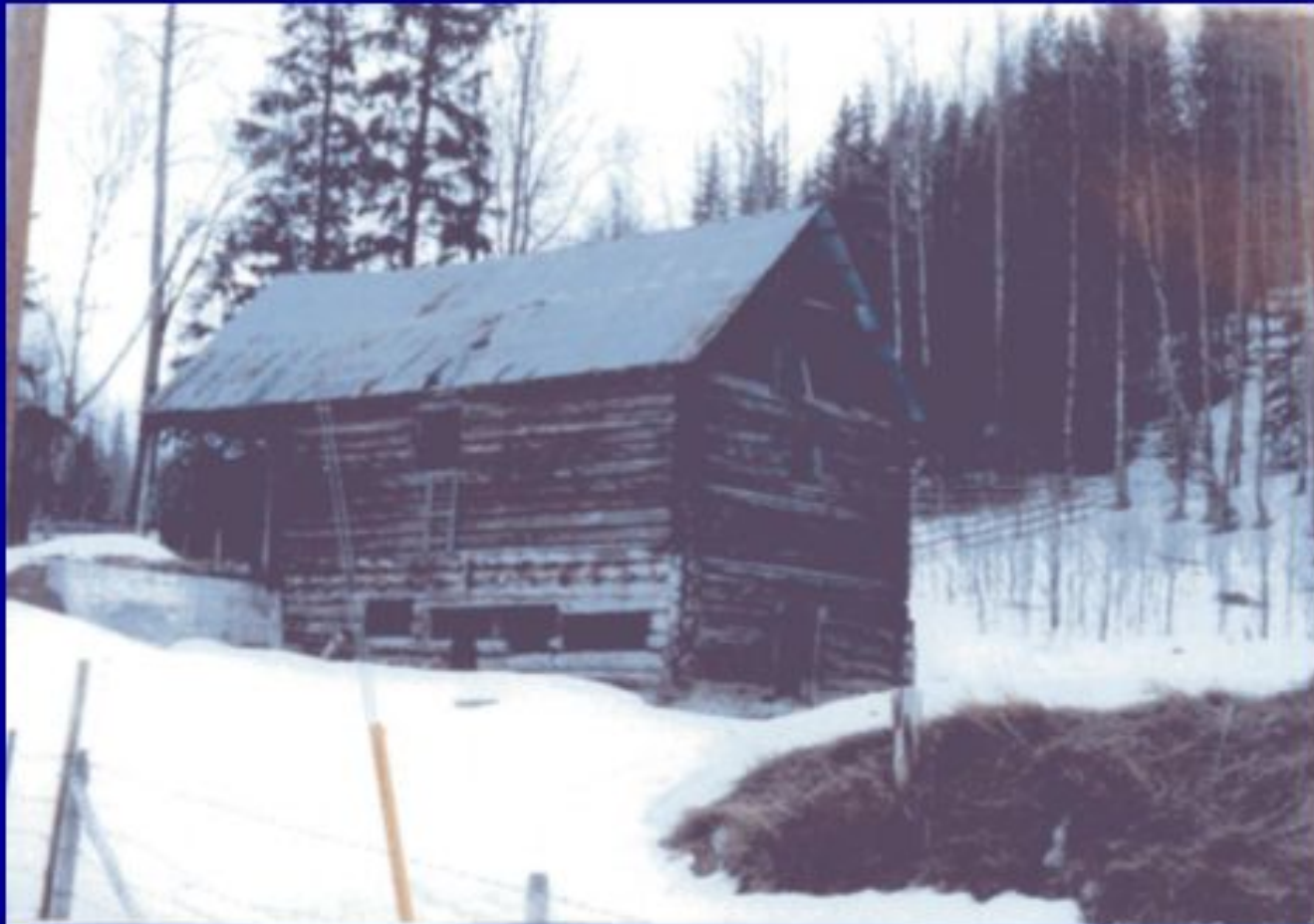
Hardy barn built by Tom Turner
