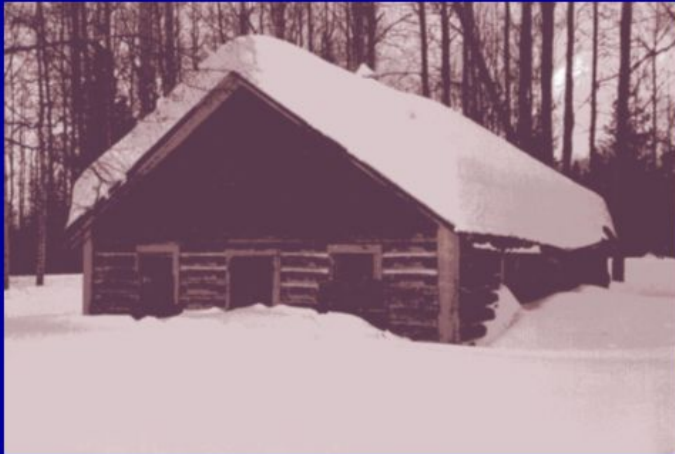
Lochyer log house before it fell down
