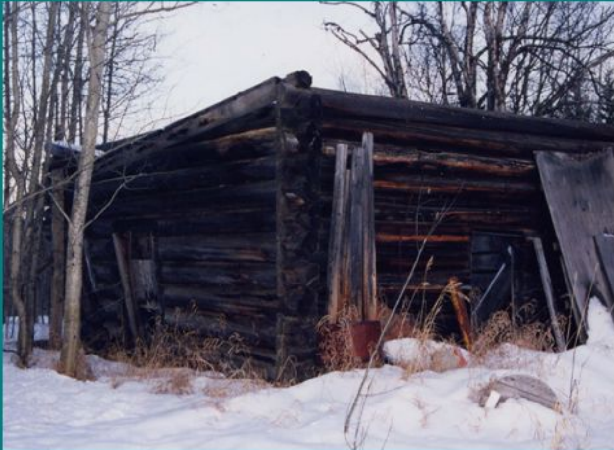
Walls of Jack Hamilton's house
